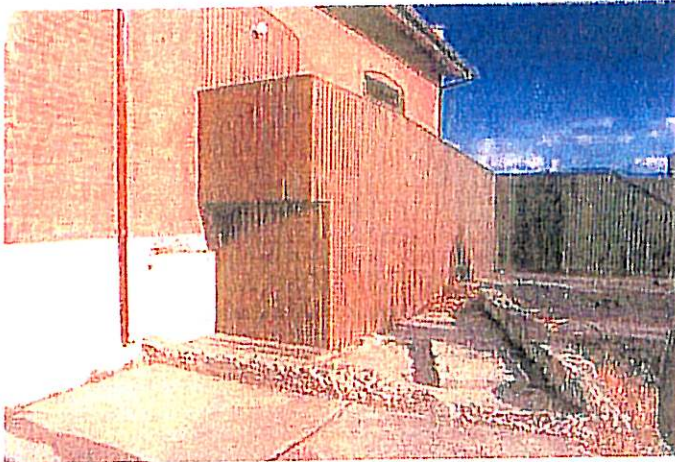
Fig 9: Concrete apron on south side showing outline of previous walls and machinery bases
