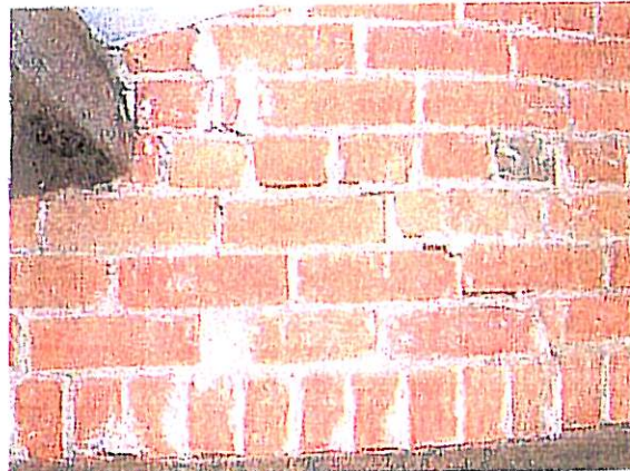
Fig 28: Cracking of Upper Level brickwork
