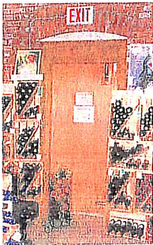
Fig. 32: Exit door blocked and incorrect panic hardware
