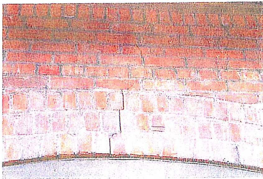
Fig 19: Example of typical cracking through brick and mortar over window opening. South elevation
