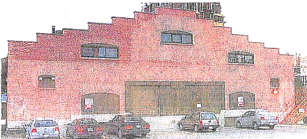
Fig 8: West elevation with different brick types indicating sections rebuilt with old (right) and modern (left) bricks during the 1983 rehabilitation
